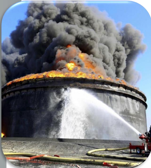
Libya Es Sider Port, Oil Tank Fire (2014)
